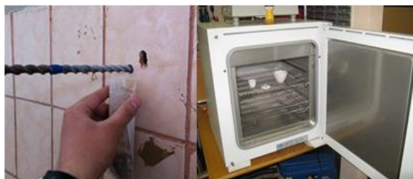
Fig. 6. Drilling and collecting of brick dust and the drying oven used for drying brick dust
